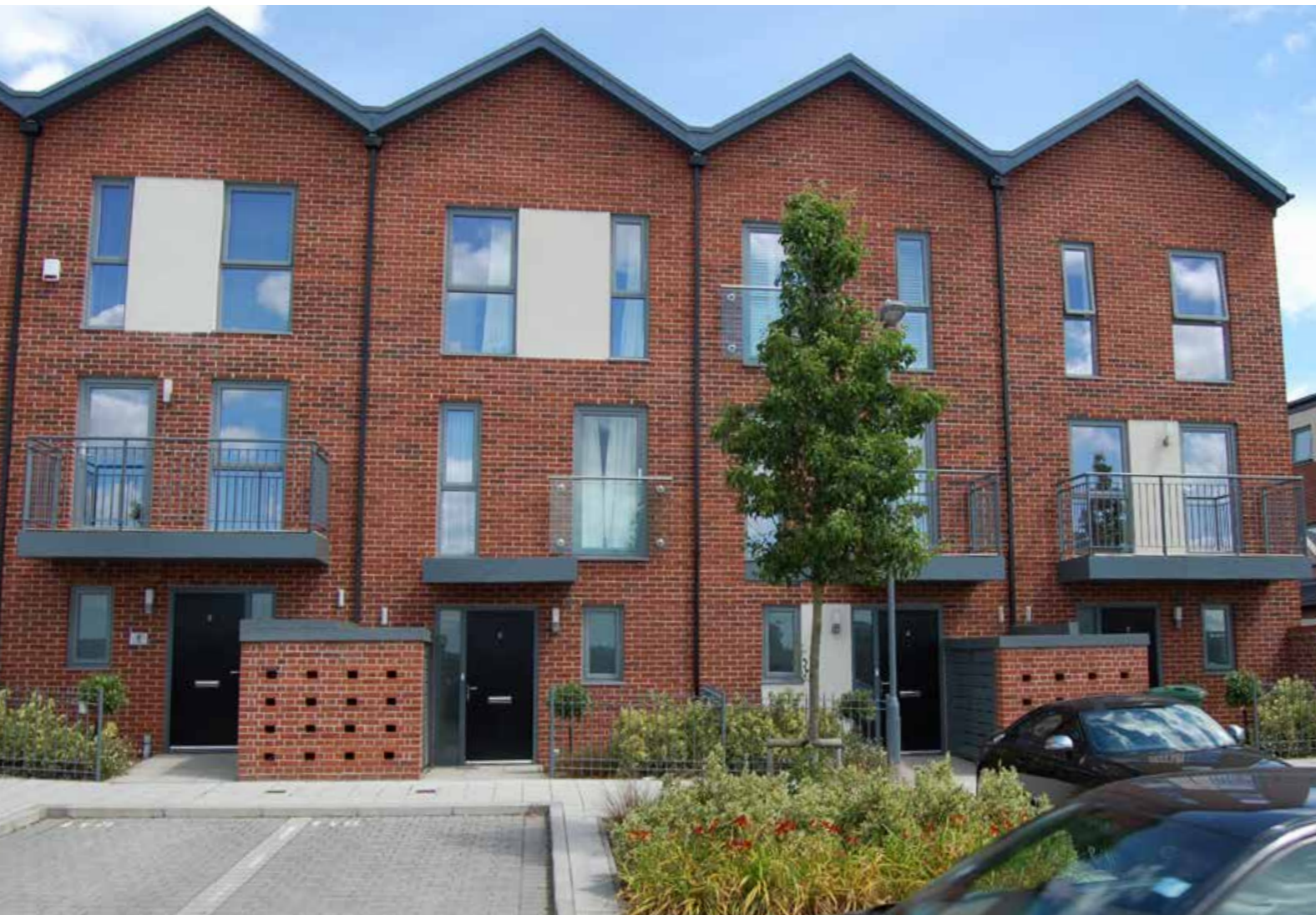
Robust brick bin stores, Centenary Quay, Southampton, Crest Nicholson
