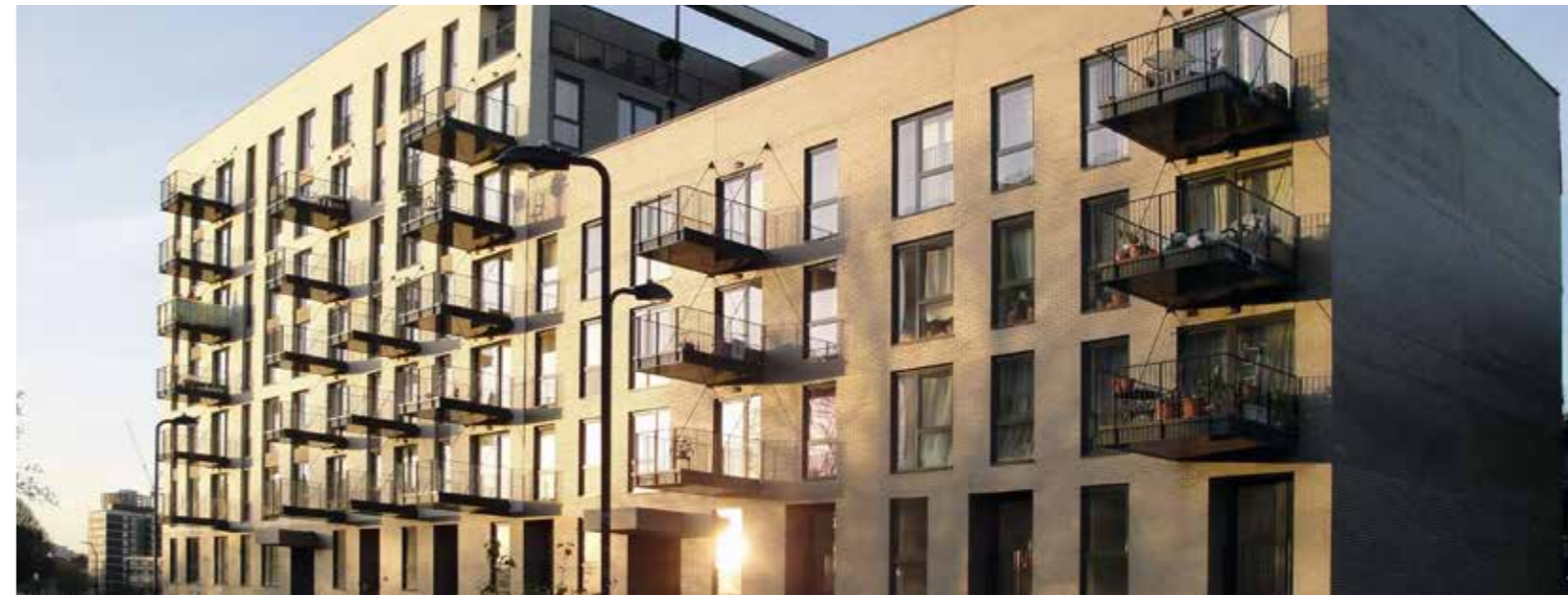
Bridport House, Hackney, London Borough of Hackney
