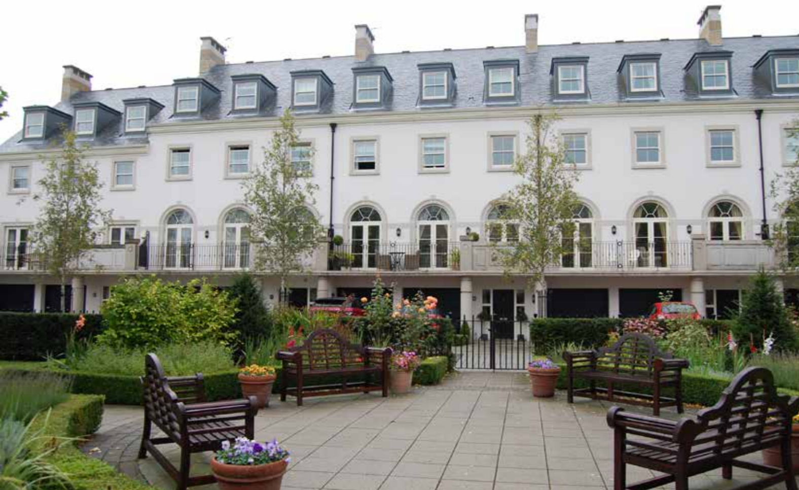
Shared garden, The Square, York, Nixon Homes
