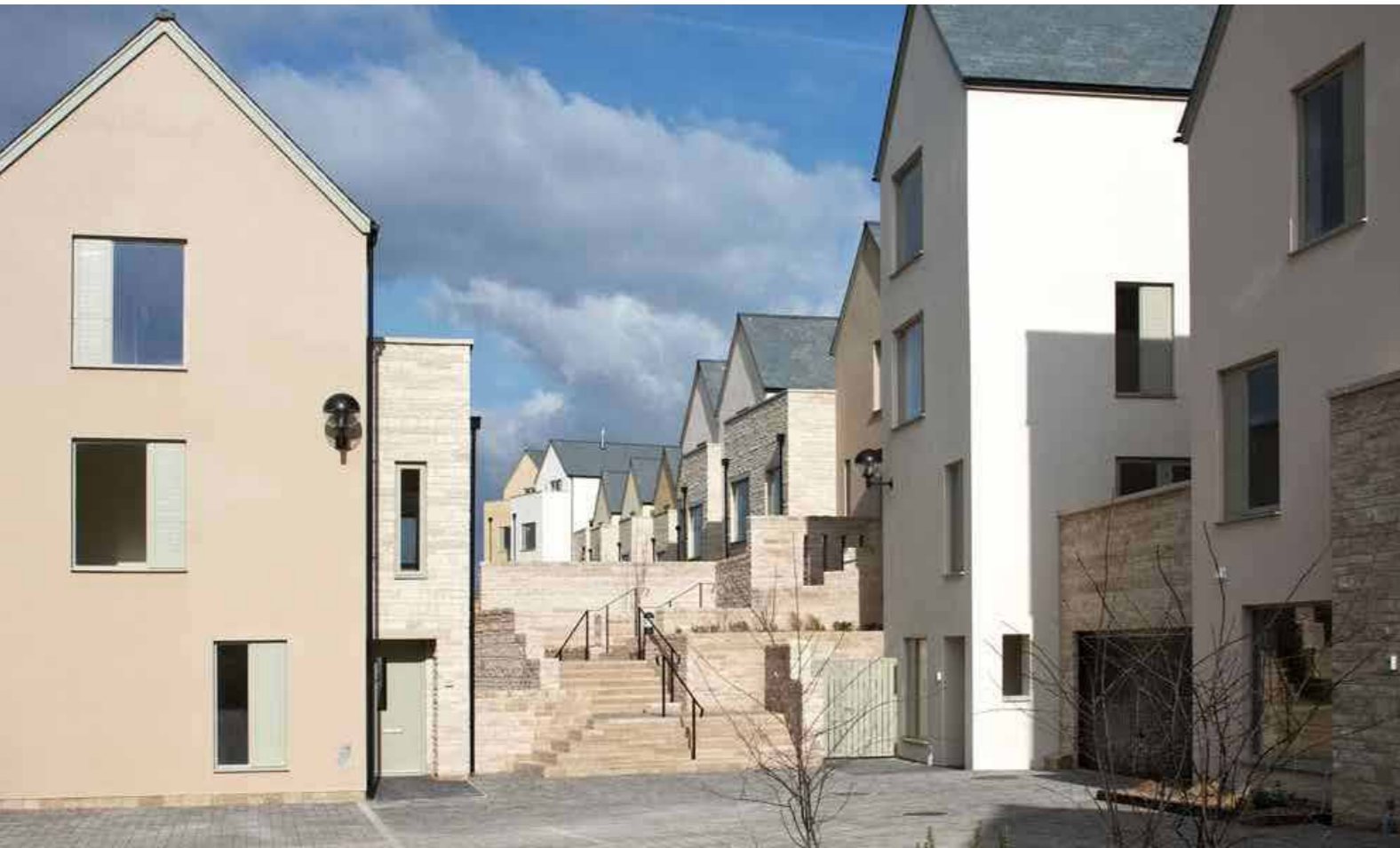
Hard landscaping is responsive to the different levels on site, Osprey Quay, Weymouth, Zero C Developments
