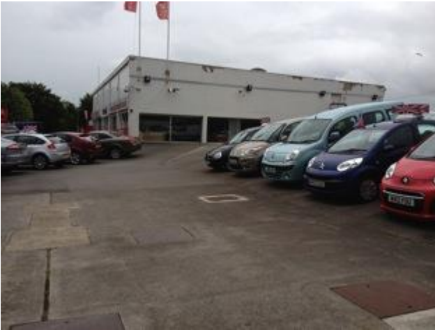
Photograph 1. Car showroom and forecourt
