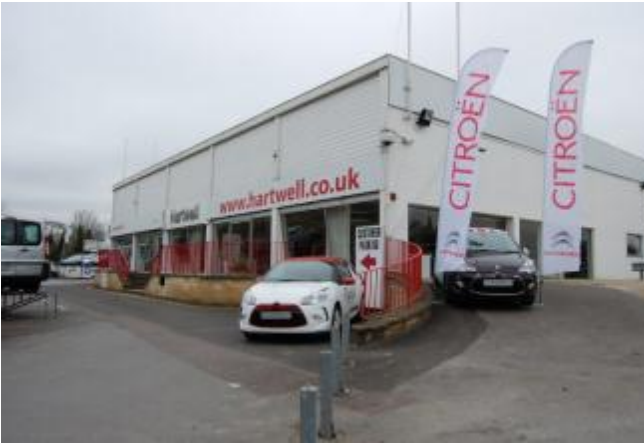
Photograph 7. Car showroom and forecourt
