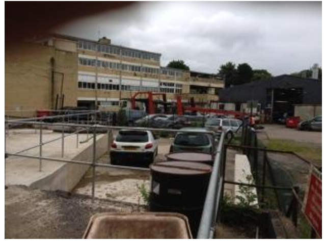
Photograph 2. View of building 1 from the rear showing the offices and undercover parking (RHS)
