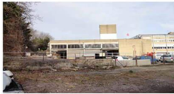
02 View looking towards the batching plant
