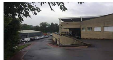
04 View looking down existing car ramp
