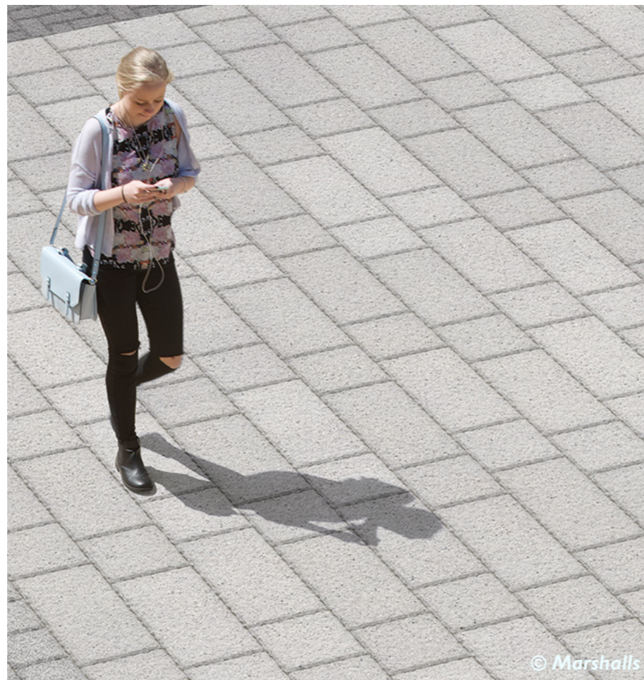
Permeable flags to key pedestrian route
