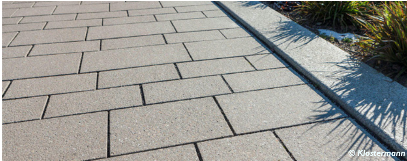
Concrete blocks to wider courtyards
