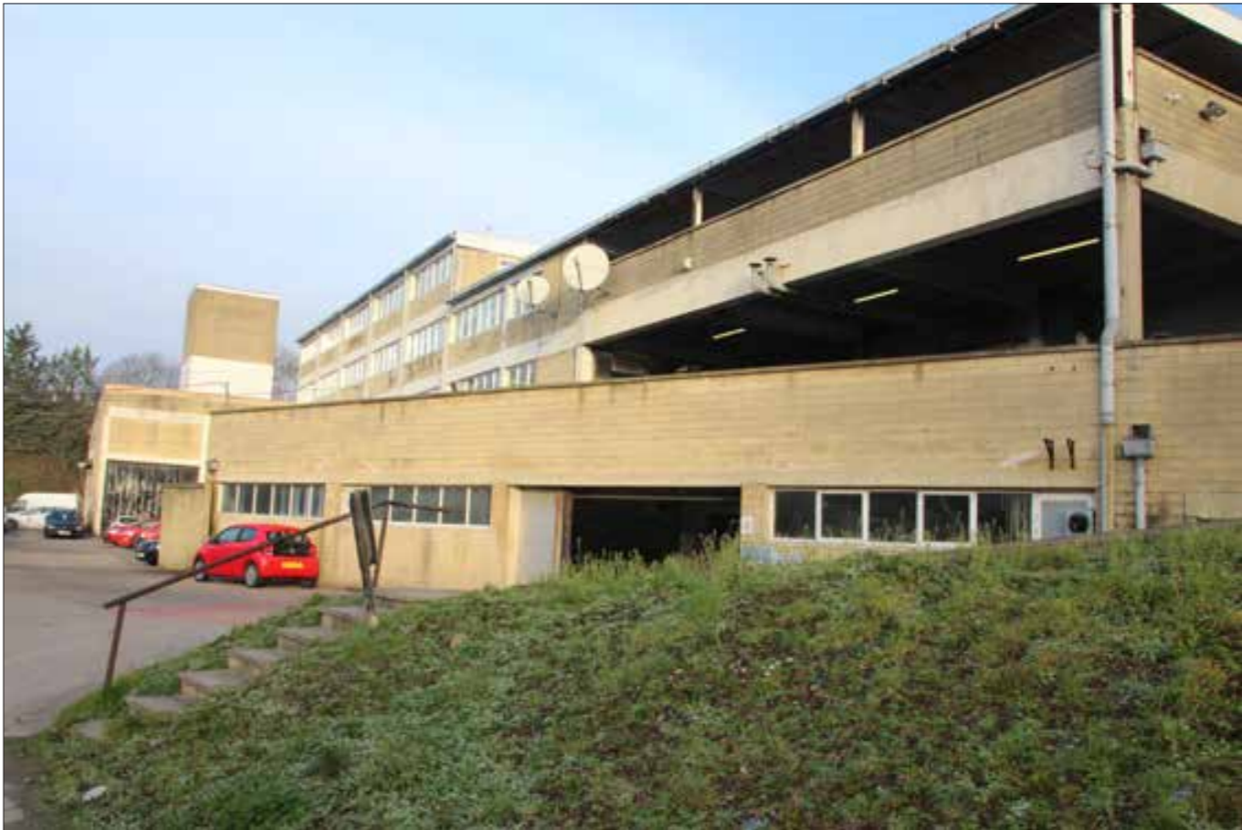
Site character view B - Southern facade of existing building.
